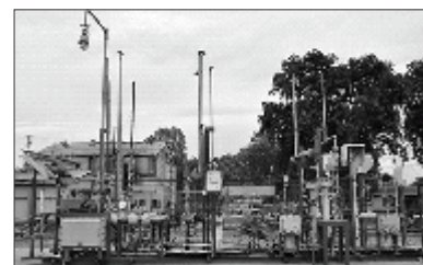
Natural Gas Plant
