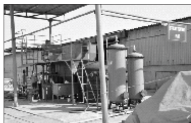
Effluent Treatment Plant
