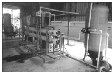
DM Water Plant
